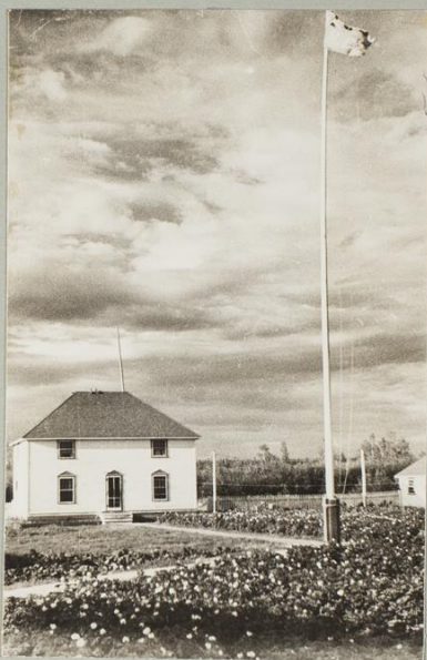
THE DWELLING HOUSE
